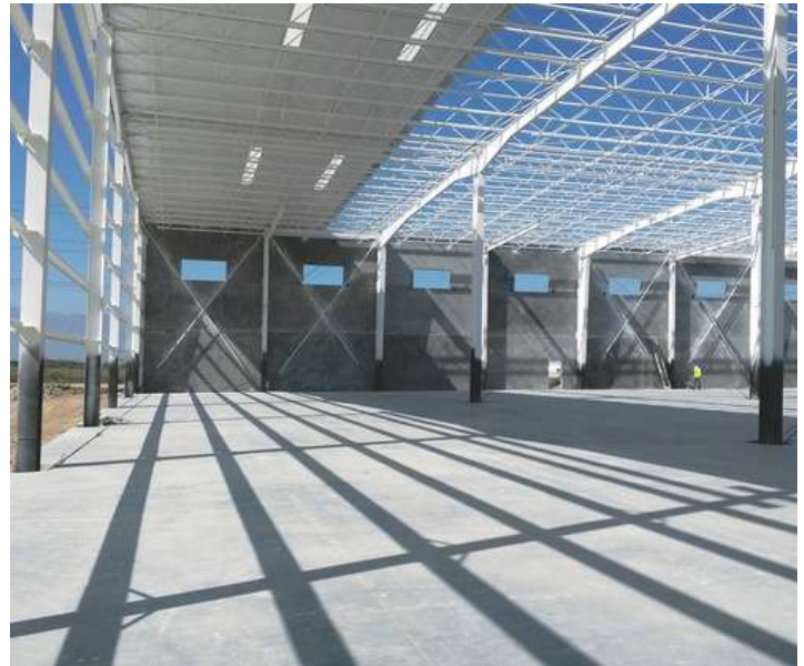
Figure 1. Ternium Steel Building Structure assembled from structural components.
